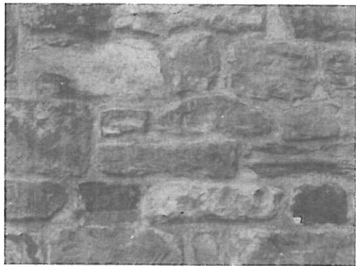
Good repointing of stonework.
