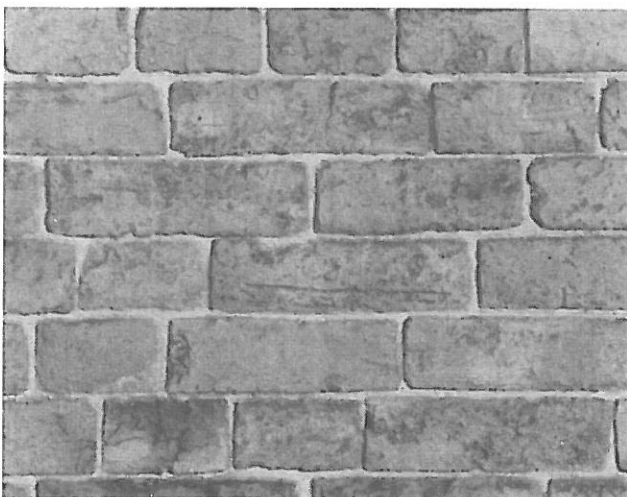
Old pointing which is sound and doesn't need repointing.
